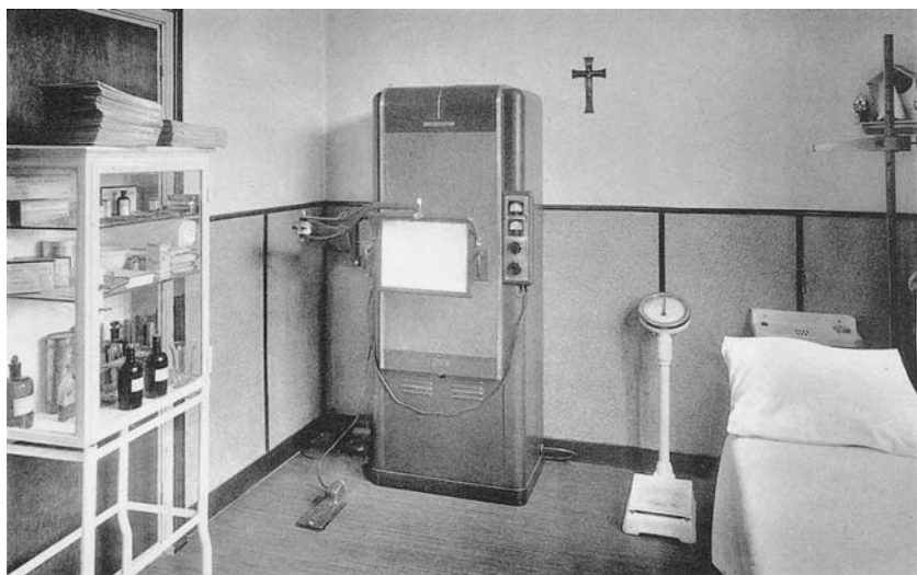
Fig. 5.6 The thorascope, the erect fluoroscopic stand for examination of the chest. Image courtesy of Dr Adrian M.K. Thomas.
